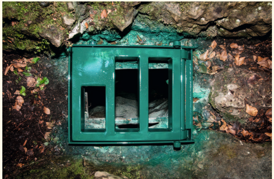
Brand new gate in Jama Ani cave. Entrance shaft is vertical, gate bars are horizontal. Picture taken from above.
