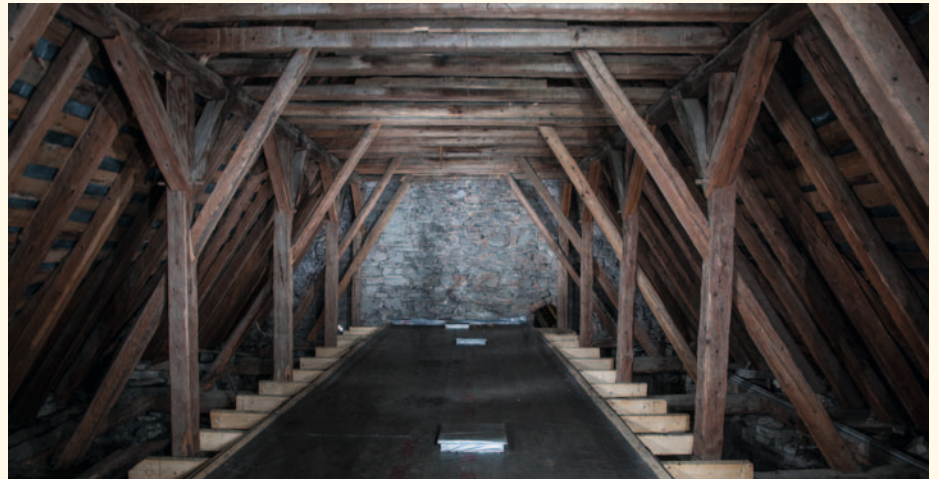
Guano platform in the Church in Łąck. Chandelier mounts are secured with foil and covered with additional roofs placed above foil.
